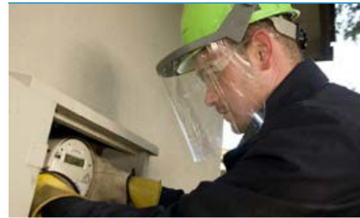
Photo Source: "Inserting SmartMeter unit" pgegreenenergy, Flickr
