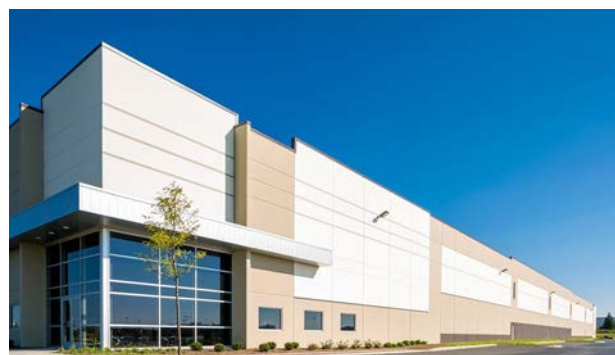
I-88 Gateway Logistics Center in Aurora
